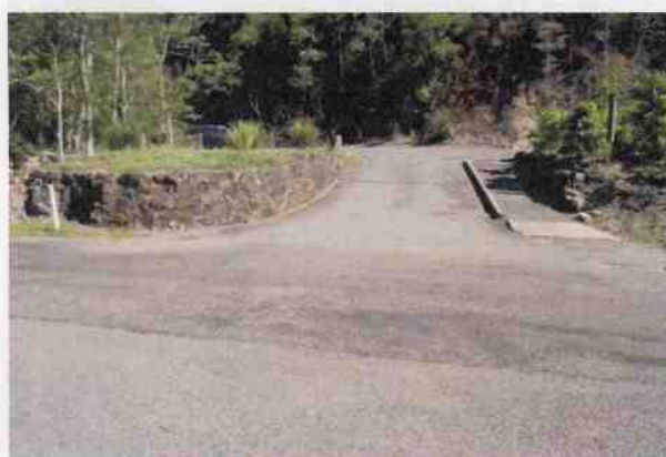
Main bridge carpark - Remnant retaining walls C303
