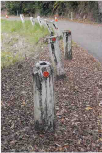
Culvert 17 - Timber guardposts & rails
