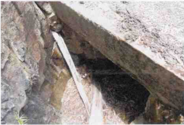
Culvert 40 - Hewn rock inlet
