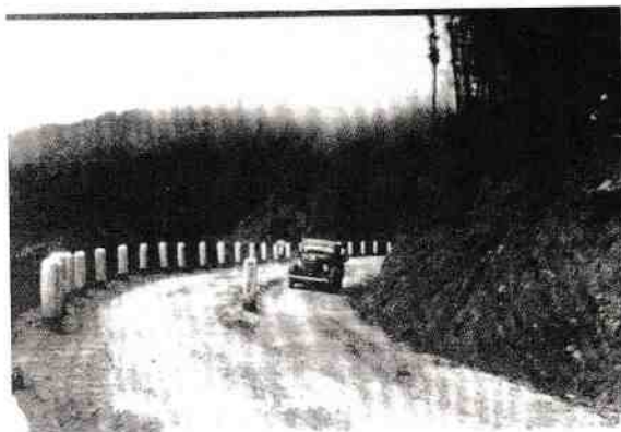
Figure 68 Early photograph showing original double tracking. Note also the extensive use of timber guardposts.
