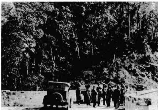
Figure 46 Governor's party inspecting the completed bridge over Little Crystal Creek. Source: City Libraries Townsville, Local History Collection No. 5006.
