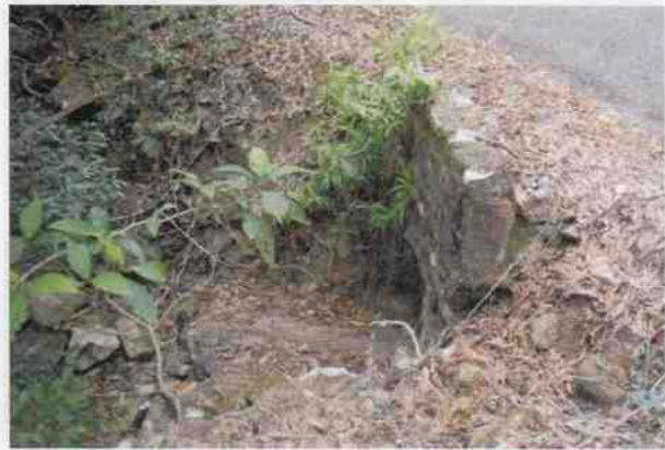
Culvert 34 - U headwall
