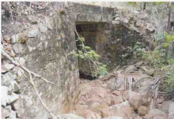
Culvert 164A - Reedy Creek B088
