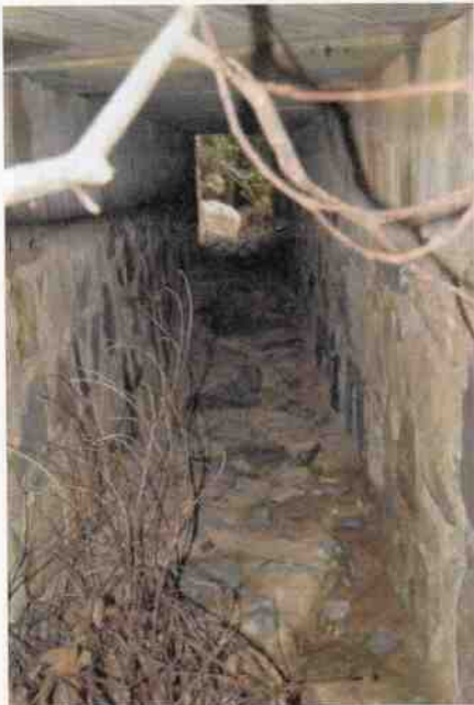
Culvert 44 - U headwall HS 2
