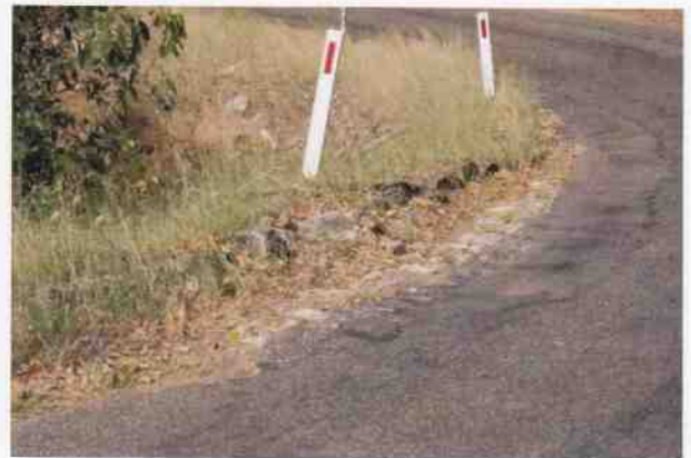
Culvert 187A - Stone kerbing and channelling
