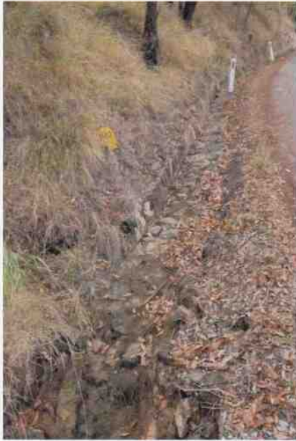
Culvert 109 - Stone kerbing & channelling B204
