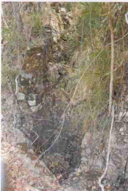
Culvert 145 - Stone training wall
