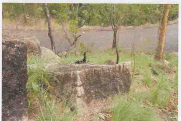
Culvert 206A - Quarry site
