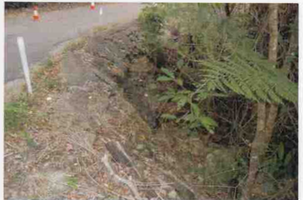
Culvert 54 - E headwall
