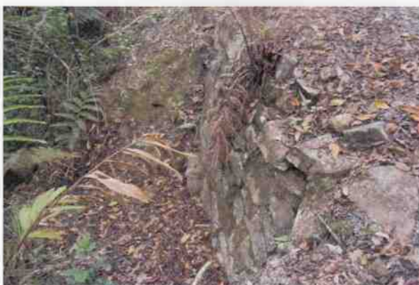
Culvert 24 - E headwall
