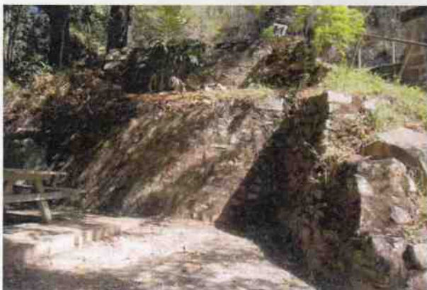
Main bridge - Stone retaining wall
