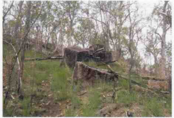
Culvert 206A - Quarry site
