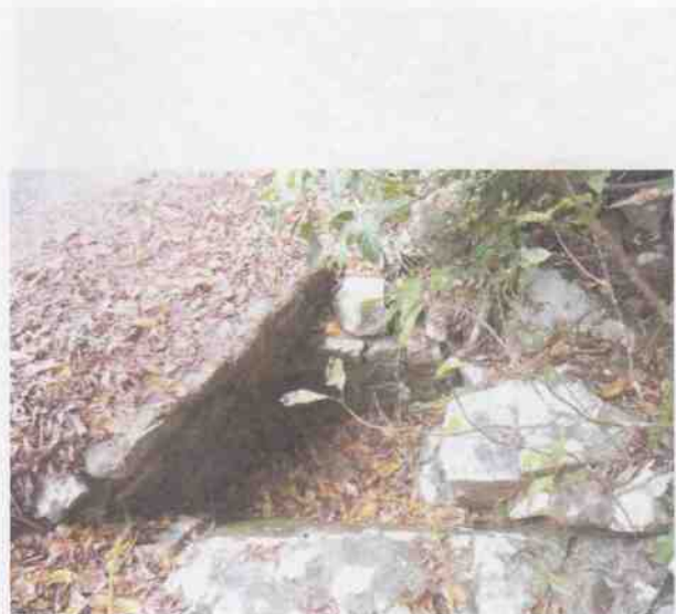
Culvert 25 - U headwall
