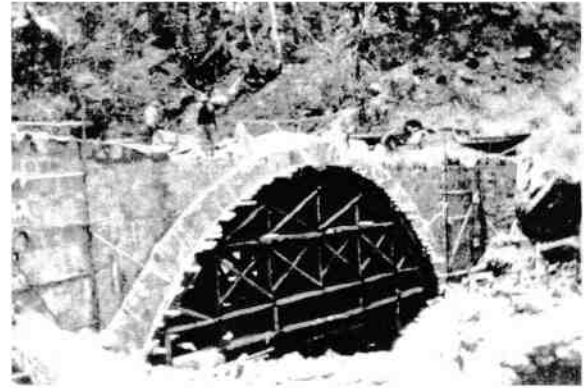
Figure 43 Bridge close to completion in 1932 Source: City Libraries Townsville, Local History Collection No. 0000/0000676.
