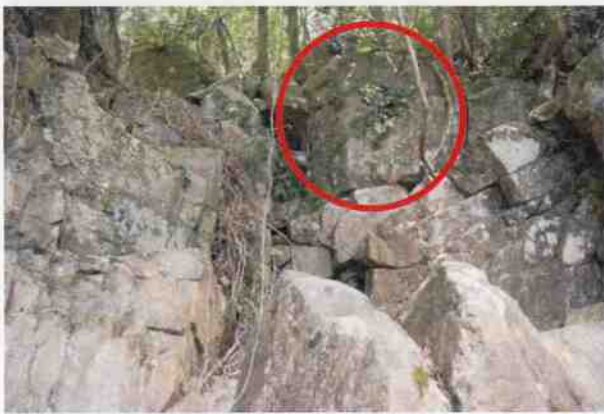
Culvert 85 - Stone training wall
