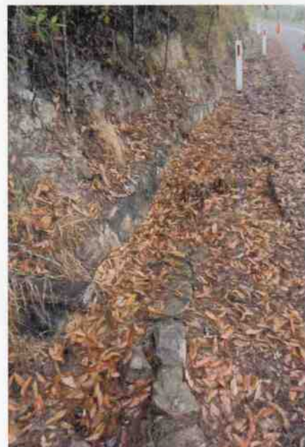
Culvert 131 - Stone kerbing & channelling
