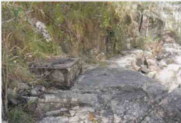
Main bridge - Stone plinth on upstream side
