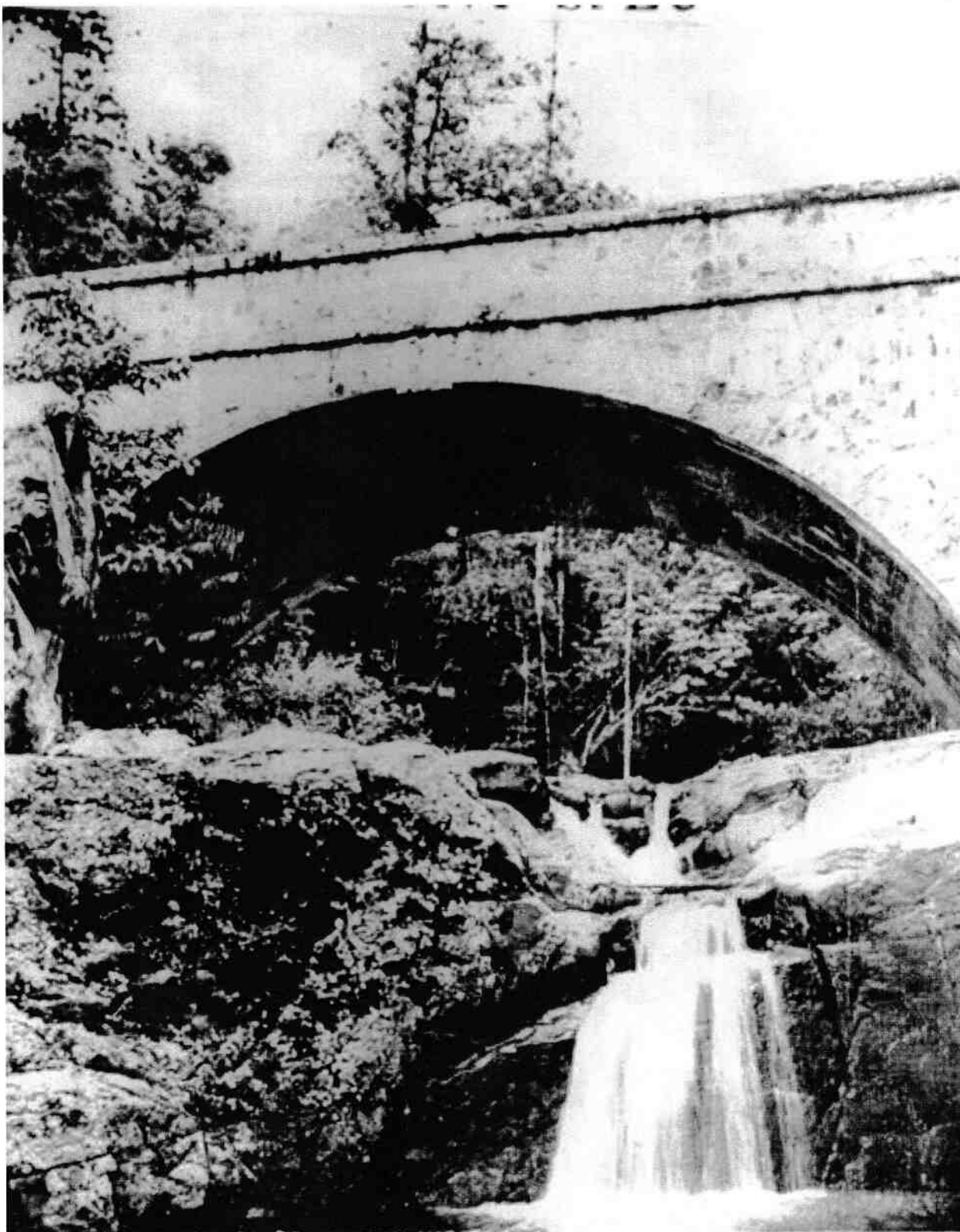
Figure 51 Bridge over Little Crystal Creek, 193? Source: City Libraries Townsville, Local History Collection No. 0007/0007036.
