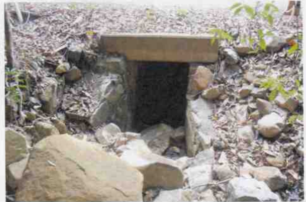
Culvert 48 - U headwall
