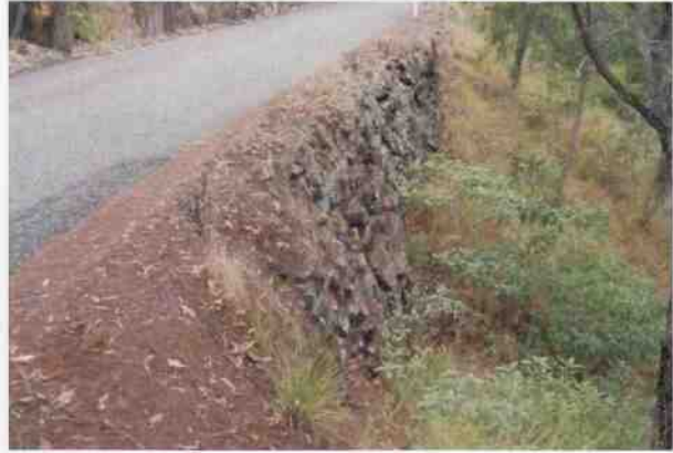
Culvert 115 - Stone retaining wall
