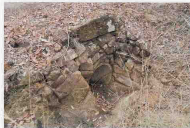
Culvert 109 - U headwall
