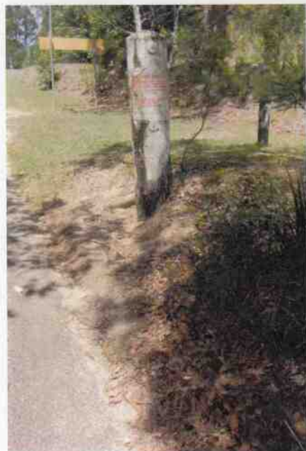
Culvert 3 – Timber guardpost
