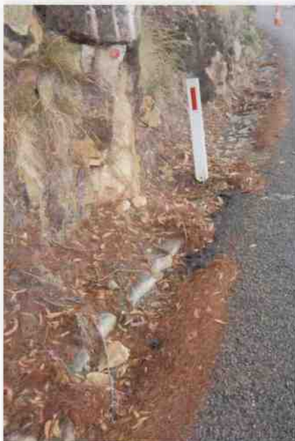
Culvert 121 – Stone kerbing and channelling
