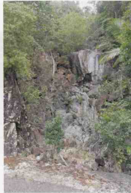
Culvert 77 – View at U
