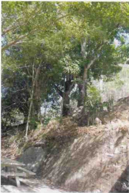
Main bridge - Stone retaining wall
