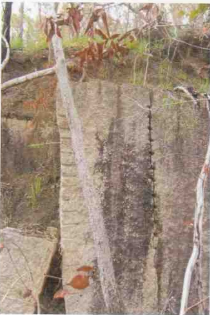
Culvert 206A - Quarry site
