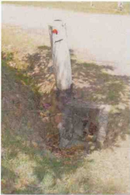
Culvert (Lennox Crescent West)
