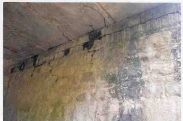
Culvert 164A B091
