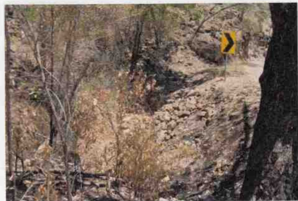
Culvert 196 - Rubble bank
