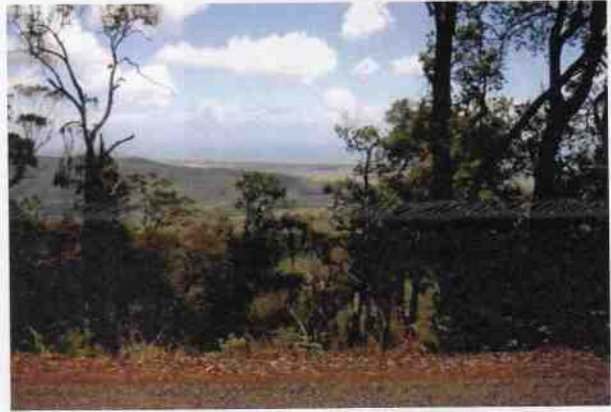
Culvert 96 - View to Halifax Bay C039
