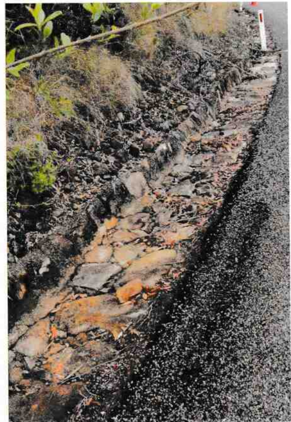
Figure 64 Stone kerbing and channelling
