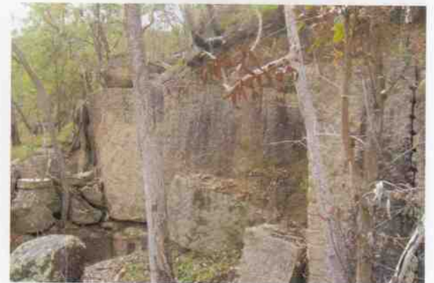
Culvert 206A - Quarry site
