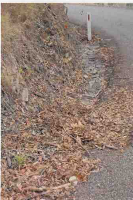
Culvert 109 - Stone kerbing & channelling
