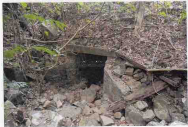
Culvert 52 - U headwall
