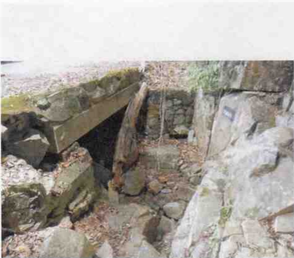
Culvert 85 - U headwall
