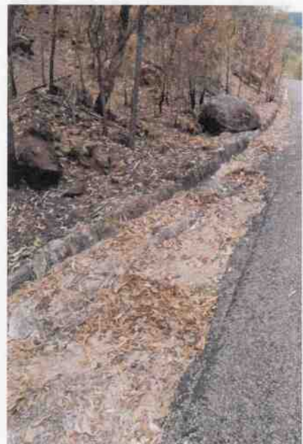
Culvert 159 - Stone kerbing & channelling
