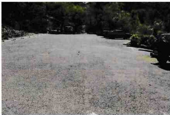
Figure 74 Existing Little Crystal Creek Bridge carpark
