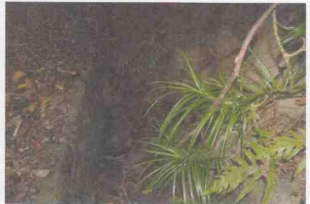
Culvert 23 - U headwall
