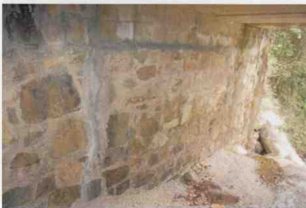
Culvert 77 - Stone retaining walls at E
