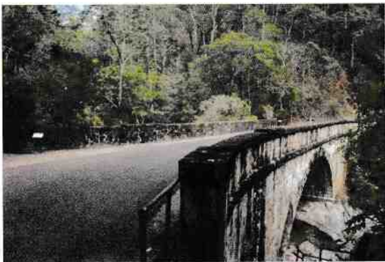
Figure 85 Little Crystal Creek Bridge
