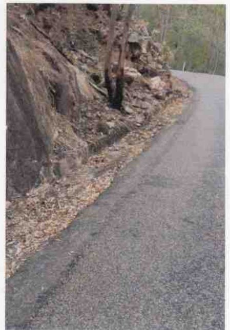
Culvert 177 - Stone kerbing
