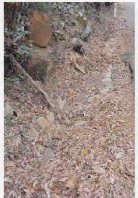
Culvert 82 - Stone kerbing & channelling
