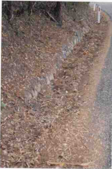
Culvert 72 - Stone kerbing & channelling C088
