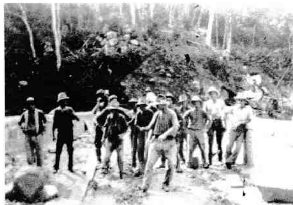
Figure 11 Workers on the bridge over Little Crystal Creek 193? Source: City Libraries Townsville, Local History Collection No. 0000/0000677.
