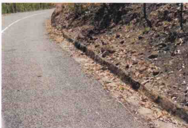
Culvert 207 - stone kerbing & channelling
