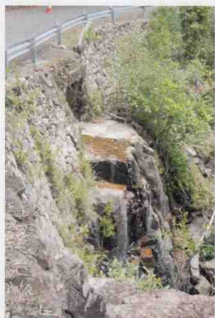
Culvert 40 - E headwall & retaining walls
