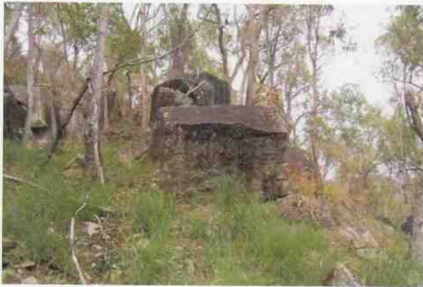
Culvert 206A - Quarry Site
