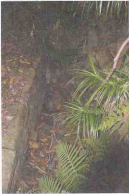
Culvert 23 - U headwall
