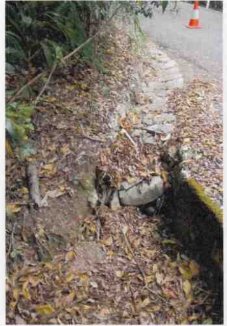
Culvert 12 - Stone kerbing & channelling C208
