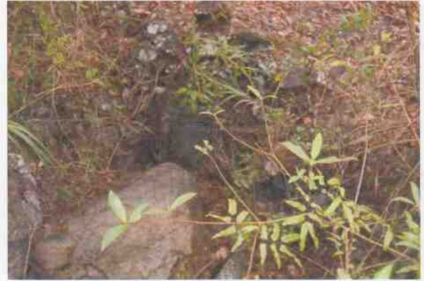
Culvert 132 - E headwall
