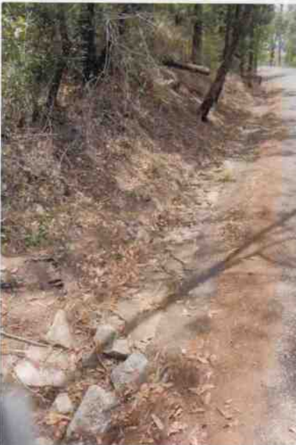
Culvert 93 - Stone kerbing & channelling
