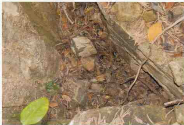
Culvert 43 - U headwall
