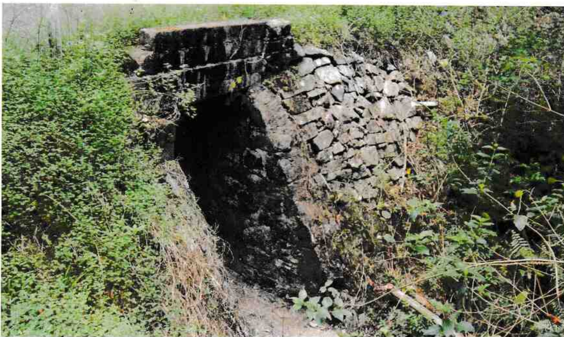
Figure 62 Large culvert headwall incorporating stone retaining wall
