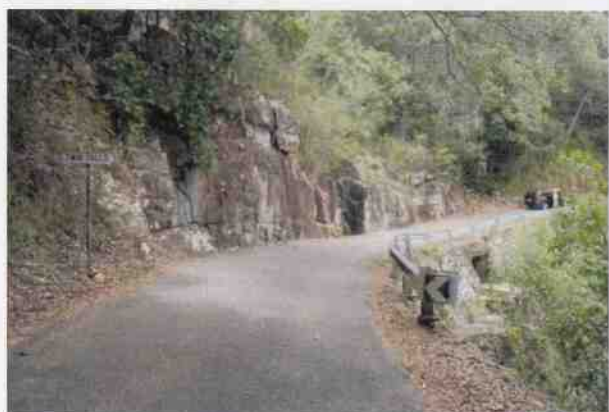
Culvert 40 - Twin Falls
