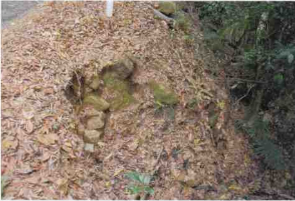
Culvert 38 - E headwall
