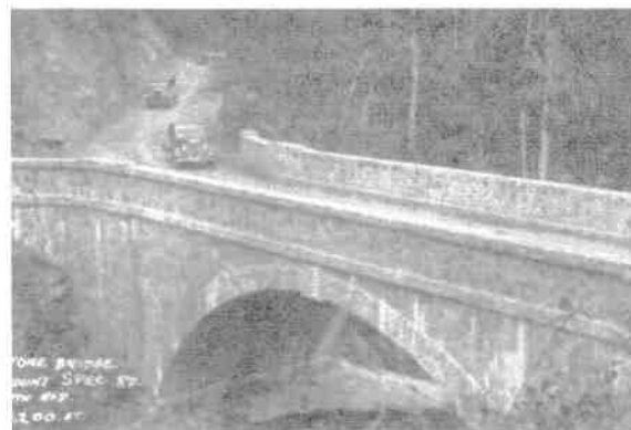
Figure 49 Completed bridge over Little Crystal Creek. Source: City Libraries Townsville, Local History Collection No. 4702.
