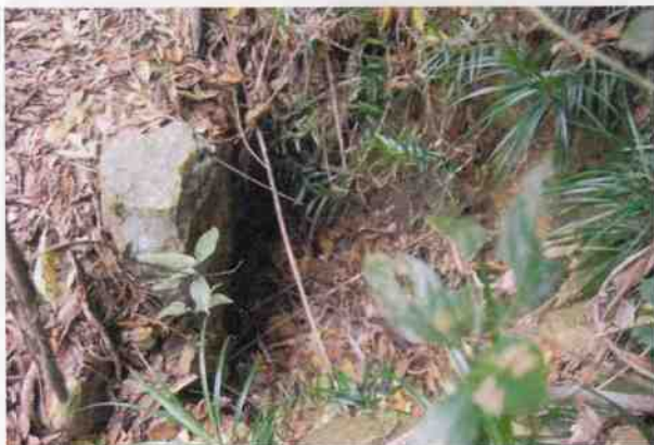
Culvert 56 - U headwall
