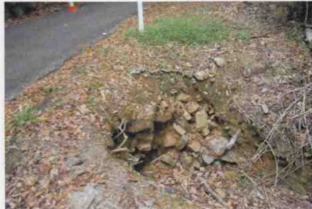
Culvert 56 - E headwall
