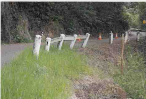
Culvert 17 - Timber guardposts & rails
