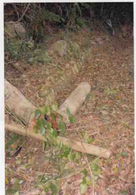
Culvert 44 - Intermittent stone channelling
