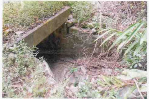
Culvert 55 - U headwall
