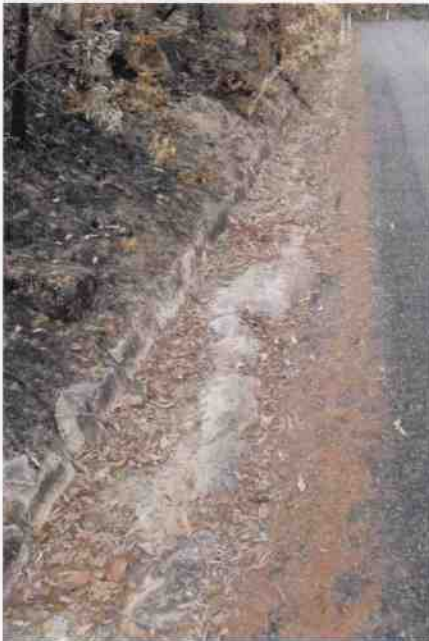
Culvert 165 - Stone kerbing & channelling B086
