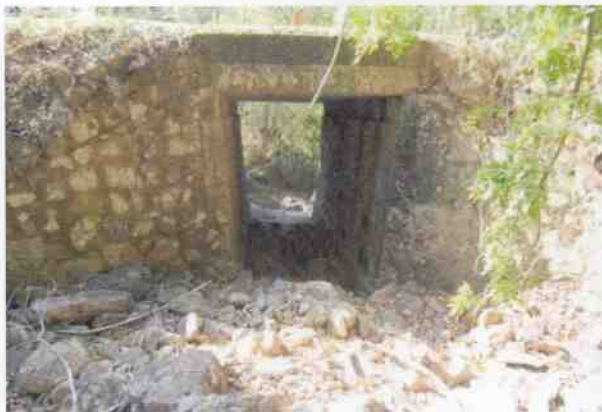
Culvert 141A - U headwall B142
