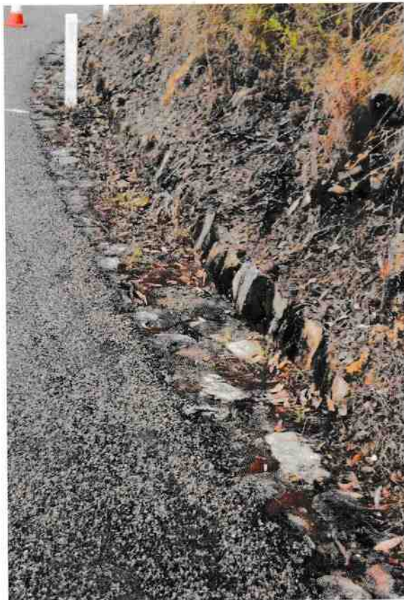
Figure 63 Stone kerbing and channelling
