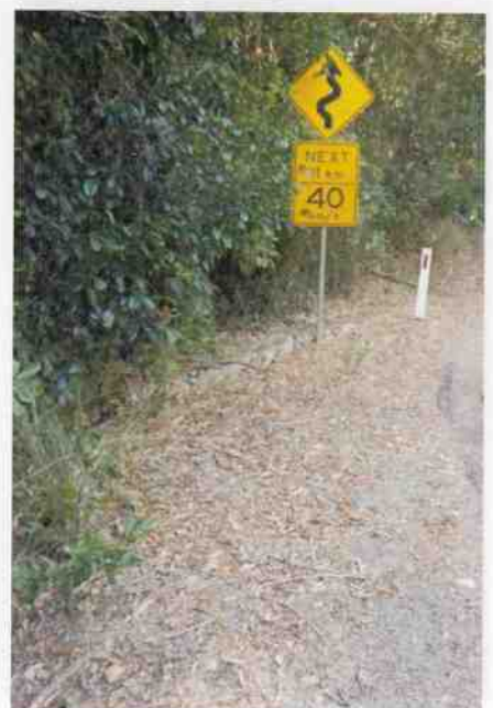
Culvert 139 – Stone kerbing
