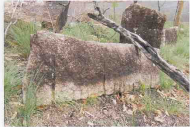
Culvert 206A - Quarry site
