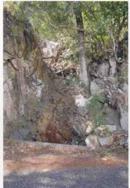
Culvert 99 - Hewn rock inlet channel
