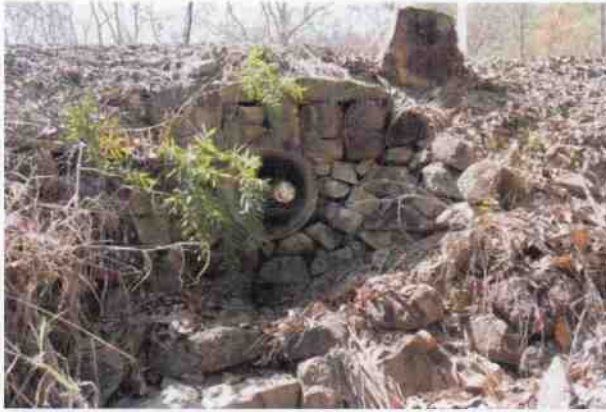
Culvert 216 - E headwall
