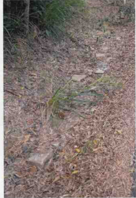
Culvert 47 - Intermittent stone channelling
