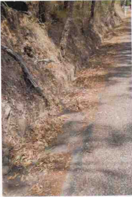
Culvert 97 - Stone kerbing & channelling C038
