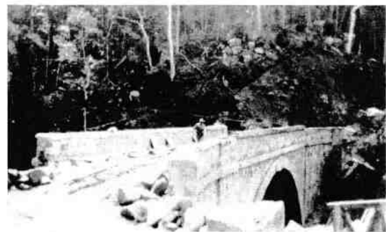
Figure 44 Bridge close to completion in 1932 Source: City Libraries Townsville, Local History Collection No. 0000/0000678.
