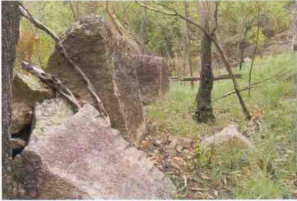
Culvert 206A - Quarry site
