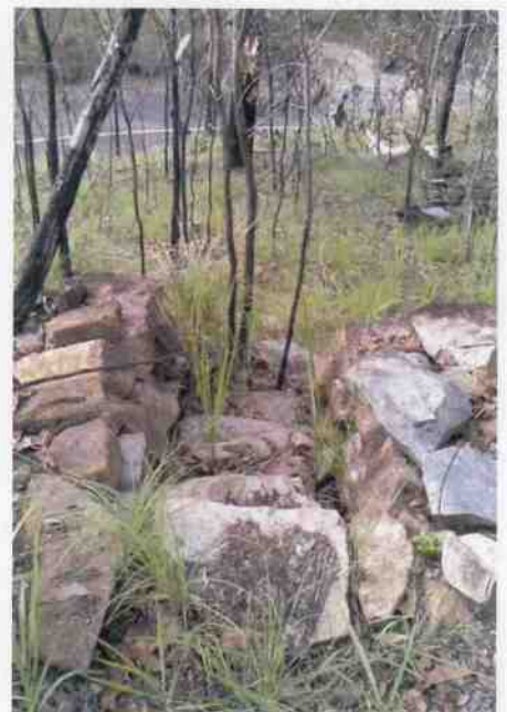
Culvert 149 - Camp site stairs
