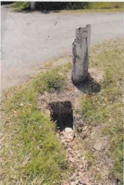
Culvert (Lennox Crescent West)
