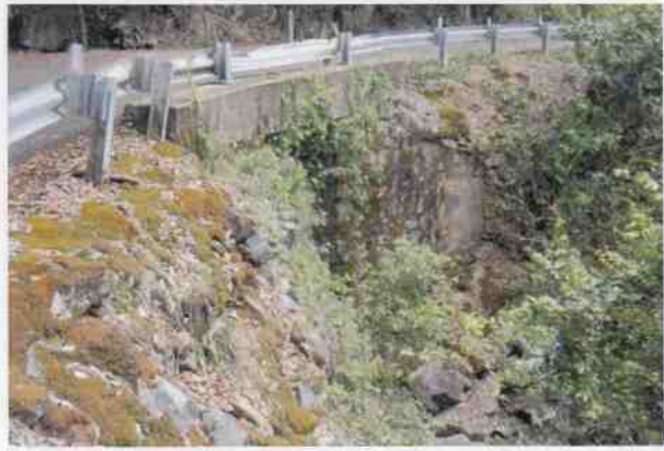
Culvert 85 - E headwall
