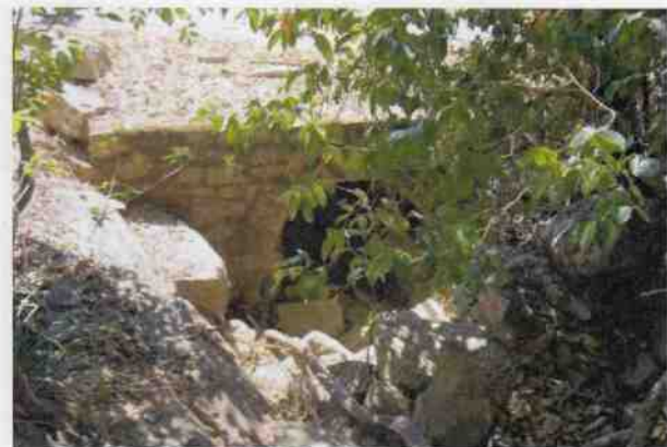
Culvert 188A - Fairy Falls
