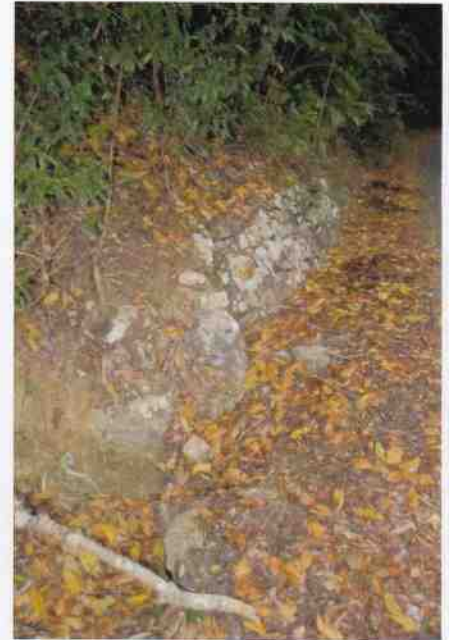
Culvert 24 – Drystone walling
