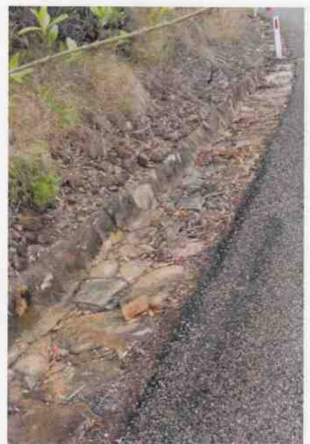
Culvert 116 - Stone kerbing & channelling
