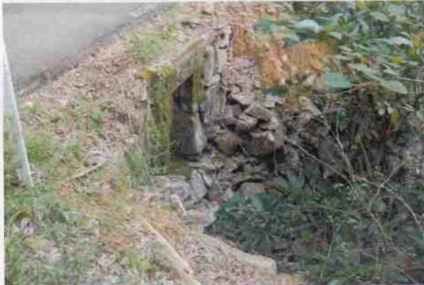
Culvert 48 - E headwall
