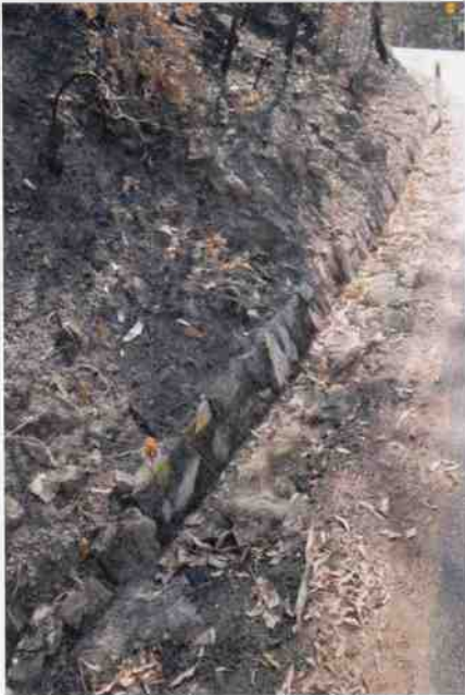
Culvert 142 - Stone kerbing & channelling B138
