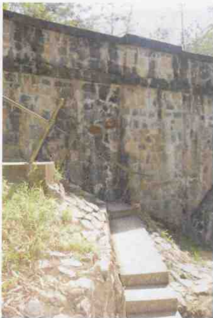
Main bridge - Concrete stairs and path
