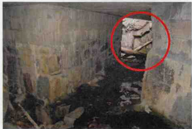
Culvert 40 - Downhill branch inlet
