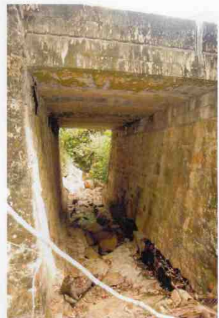
Culvert 164A B089
