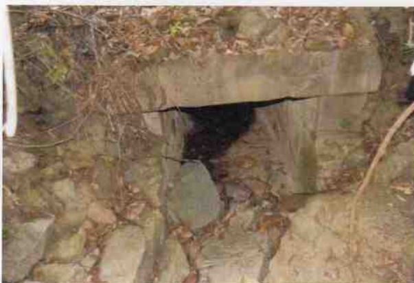
Culvert 54 - U headwall
