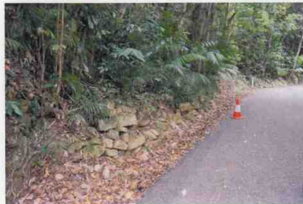
Culvert 56 - Drystone walling
