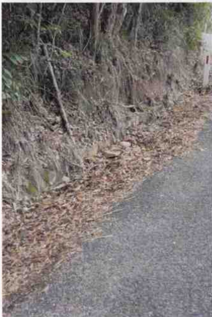
Culvert 79 – Stone kerbing & channelling
