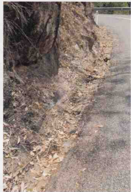
Culvert 158A - Stone kerbing & intermittent stone channelling
