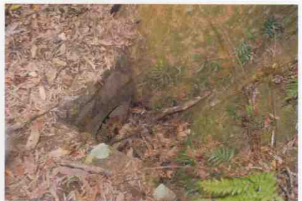
Culvert 37 - U headwall
