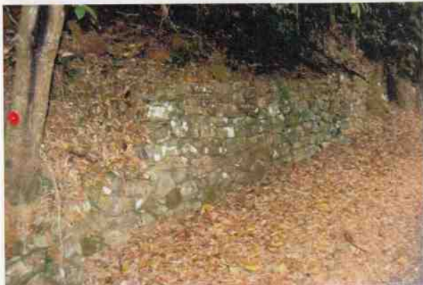
Culvert 44 - Drystone walling
