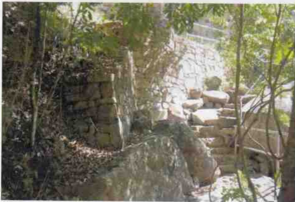
Main bridge - Stone retaining wall
