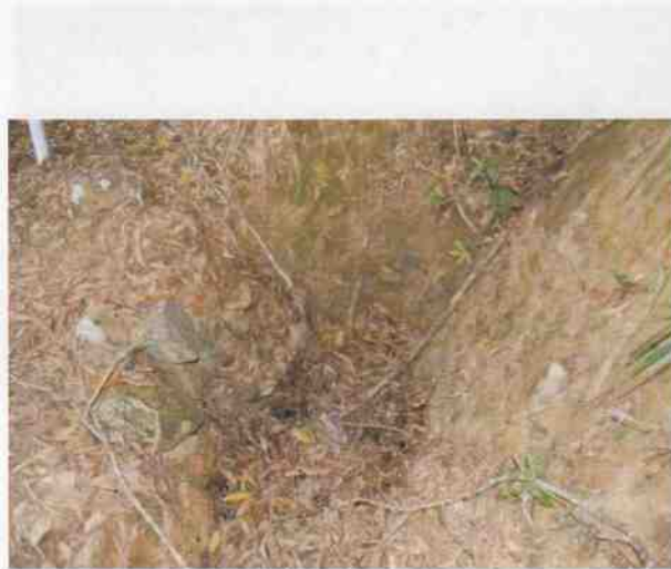
Culvert 62 - U headwall
