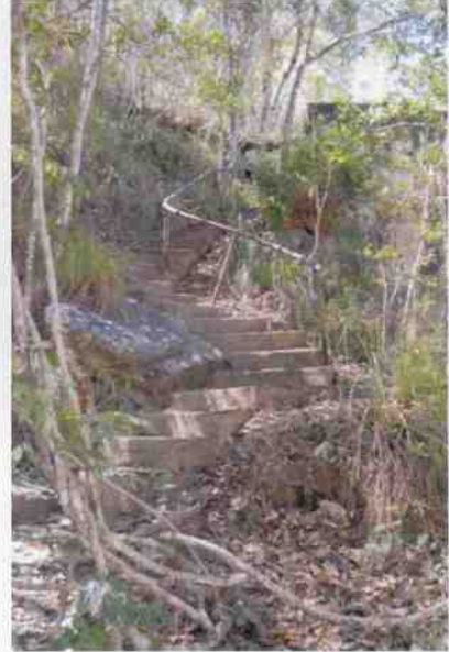
Main bridge - Concrete stairs & railing
