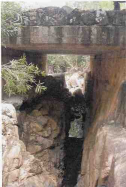
Culvert 163A - Noah's Ark Creek
