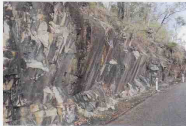
Bartlett's Bluff – large cutting between Culverts 120 and 119
