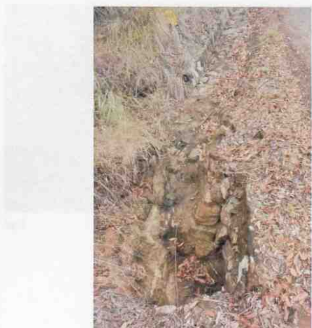
Culvert 109 - Stone kerbing & channelling
