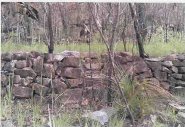
Culvert 149 - Camp site retaining wall
