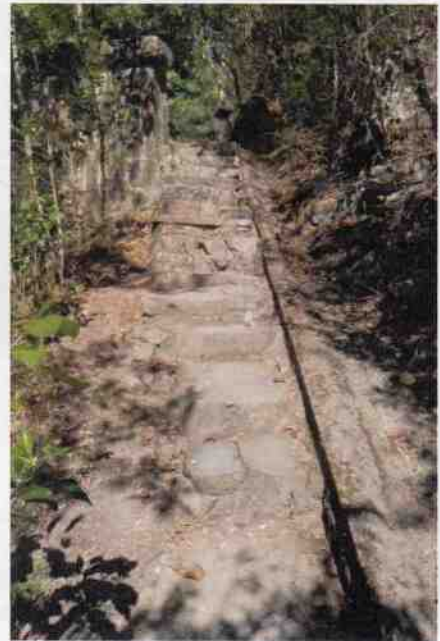
Main bridge - Stone stairs
