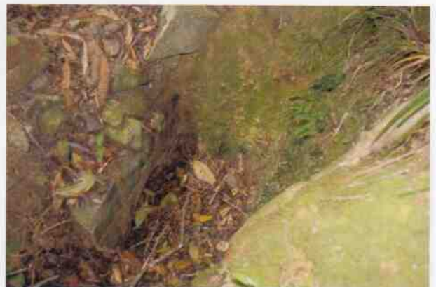
Culvert 22 – U headwall
