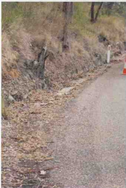
Culvert 108 - Stone kerbing & channelling B206
