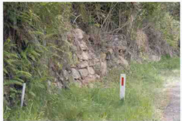
Culvert 95 - Drystone walling C044
