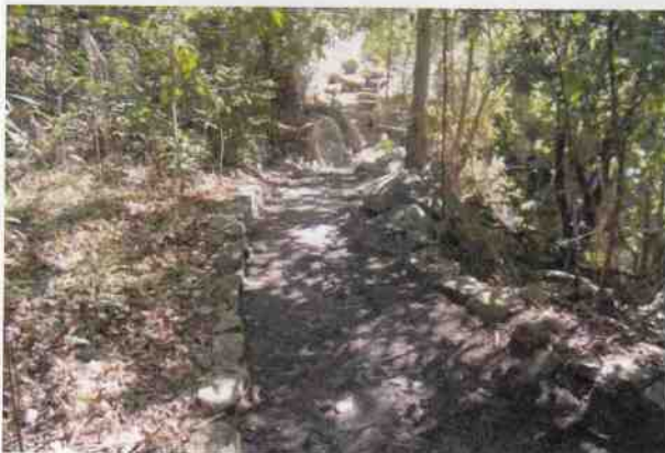
Main bridge - Stone stairs and path to lower picnic area
