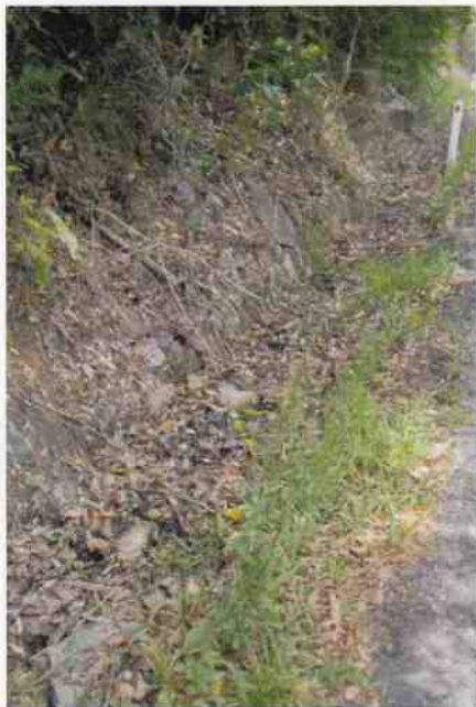
Culvert 95 - Stone kerbing & channelling C042
