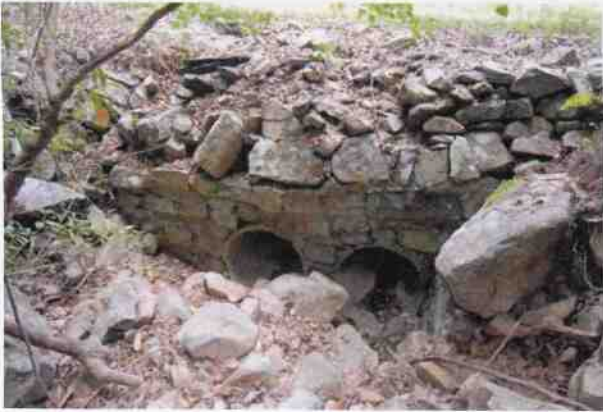
Culvert 94 - U headwall
