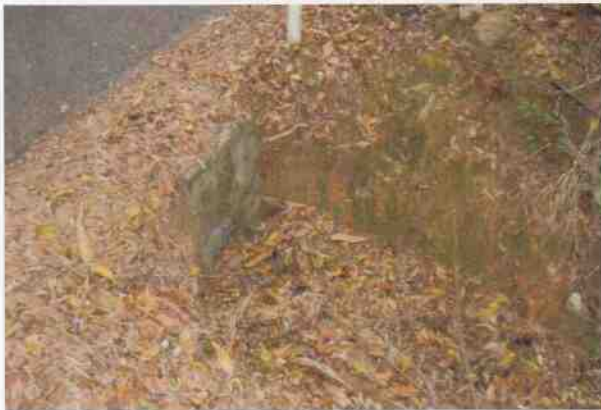
Culvert 46 - E headwall
