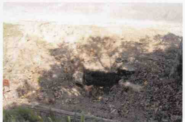
Culvert (72 Mt Spec Road)
