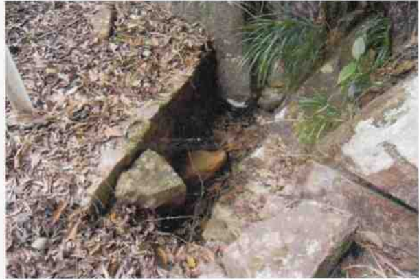
Culvert 58 - U headwall
