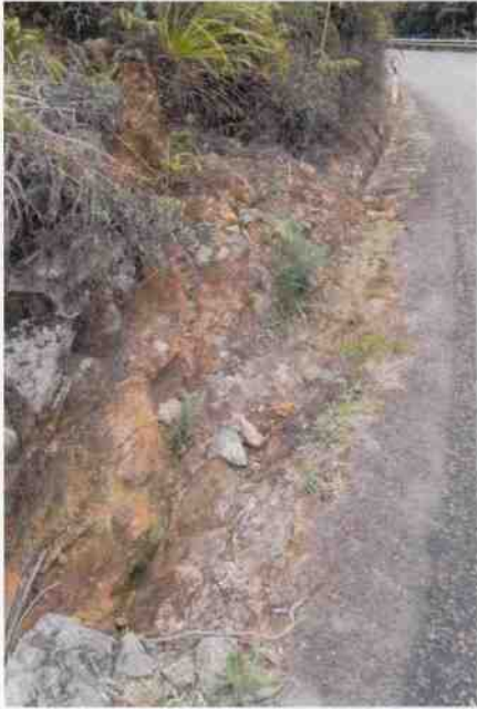
Culvert 14 - Stone kerbing & channelling C204
