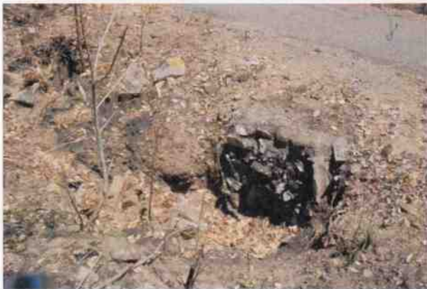
Culvert 207 - U headwall
