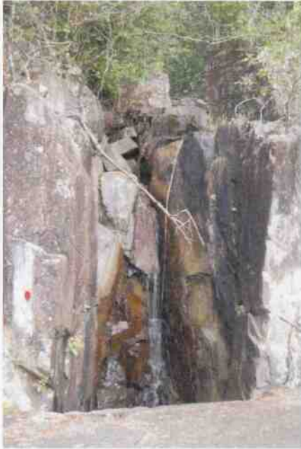
Culvert 40 - Hewn rock inlets
