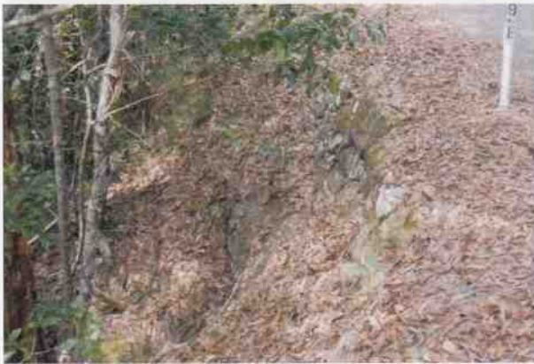
Culvert 79 – E headwall and stone retaining wall
