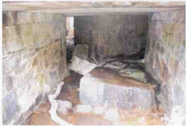
Culvert 40 - Natural rock invert
