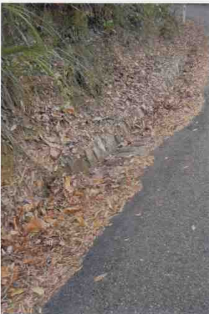
Culvert 38 - Stone kerbing & channelling
