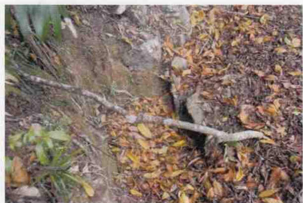
Culvert 24 - U headwall
