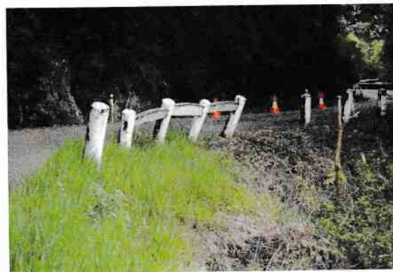
Figure 69 Surviving timber guardposts and rails uphill from Culvert 17
