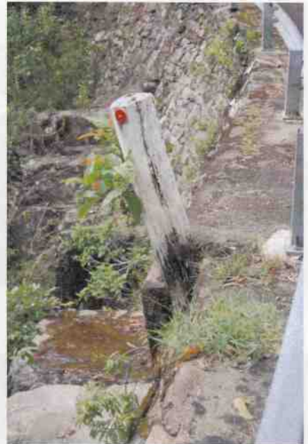
Culvert 40 - Timber guardpost
