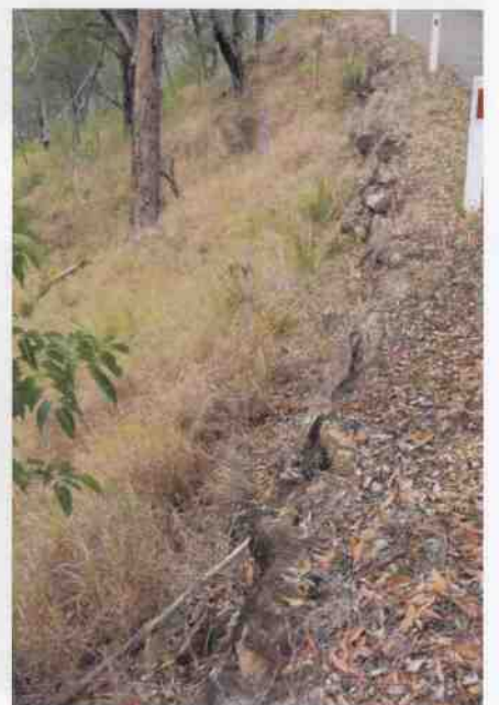
Culvert 107 - Stone retaining wall B208
