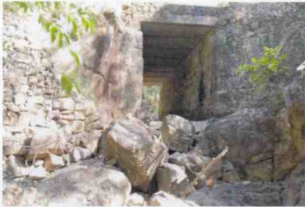
Culvert 141A - E headwall
