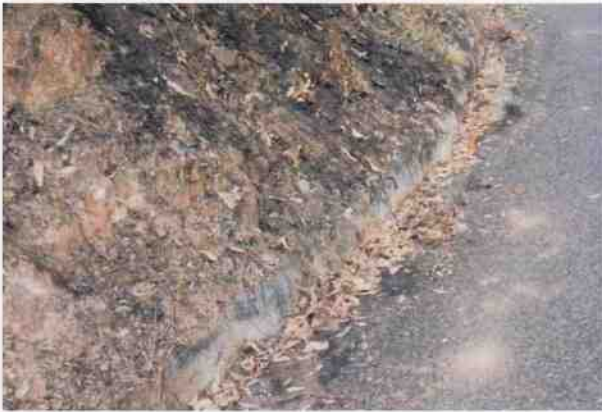
Stone kerbing & channelling between Culverts 175 and 174 B074
