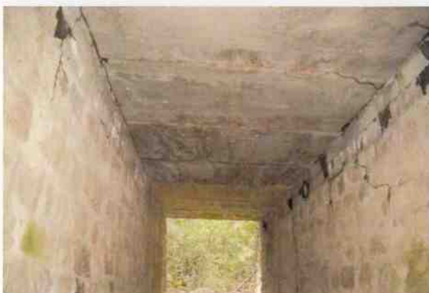
Culvert 164A B090
