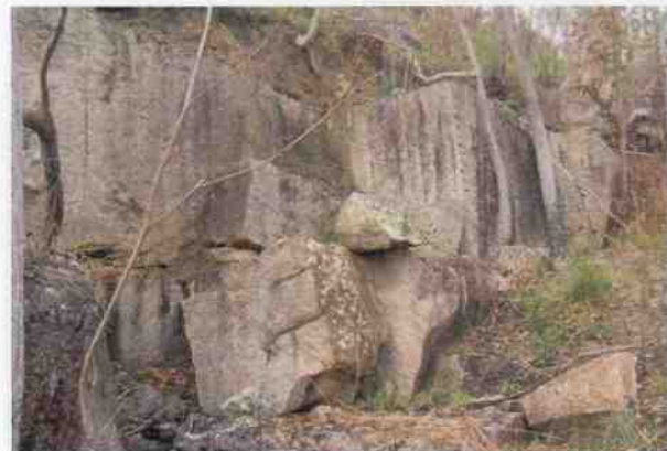
Culvert 206A - Quarry site
