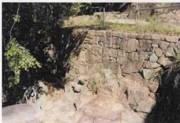
Main bridge - Stone retaining wall
