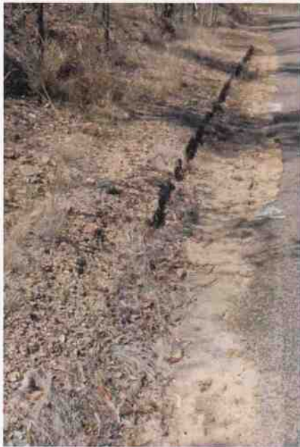
Culvert 216 - stone kerbing & channelling
