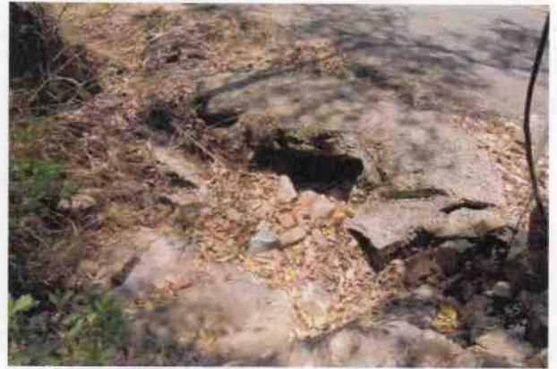
Culvert 157 - U headwall
