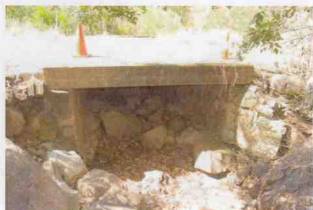
Culvert 187A - Fairy Falls
