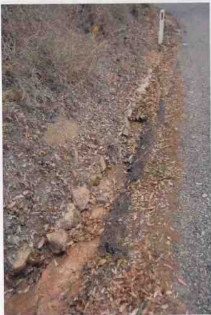
Culvert 96 - Intermittent stone channelling C040
