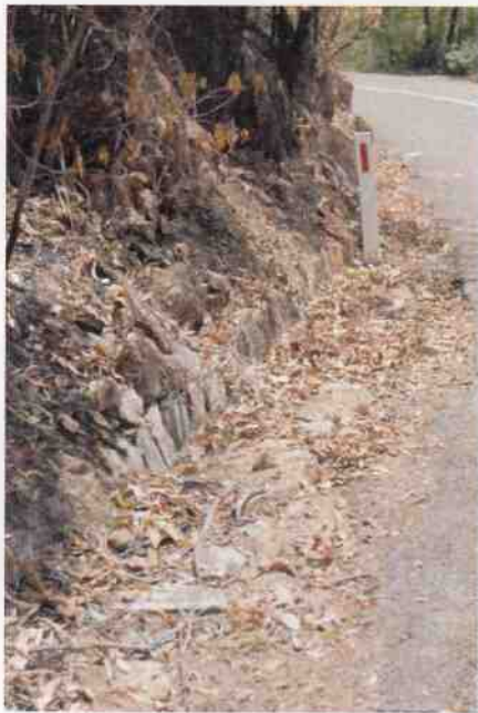
Culvert 157 - Stone kerbing & channelling
