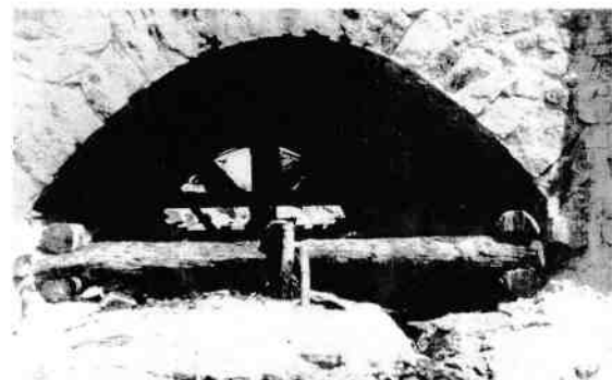
Figure 45 Completed bridge in 1932 Source: City Libraries Townsville, Local History Collection No. 0000/0000680.
