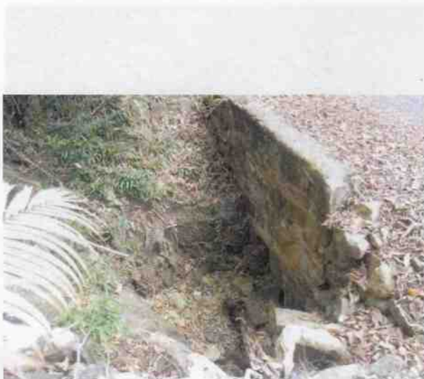
Culvert 34 - E headwall
