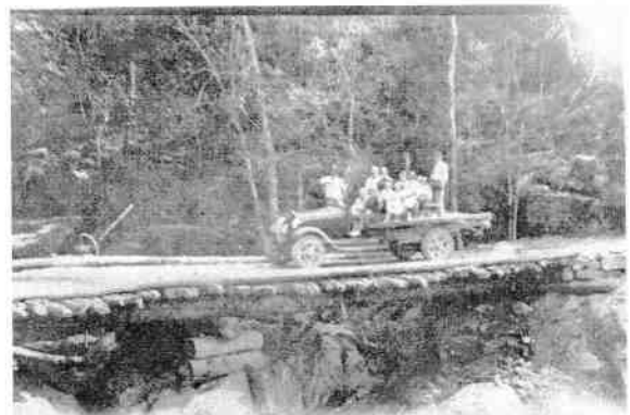
Figure 30 A Ford truck crossing the temporary timber bridge over Little Crystal Creek Bridge in 1933 Source: City Libraries Townsville, Local History Collection No. 0000/0000670
