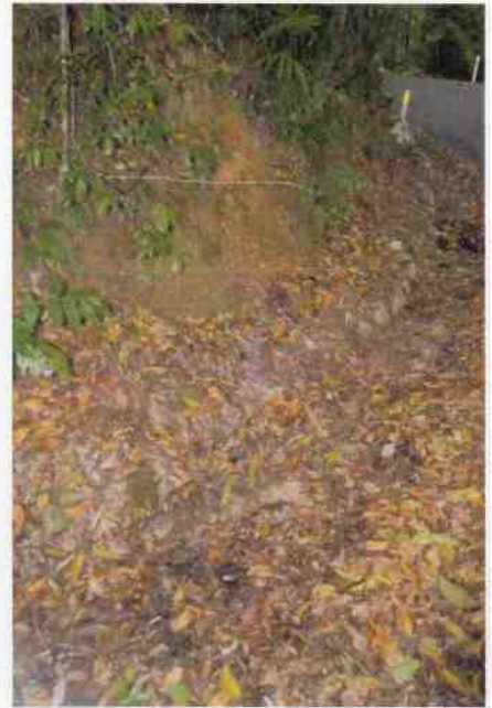
Culvert 19 - Stone kerbing & channelling
