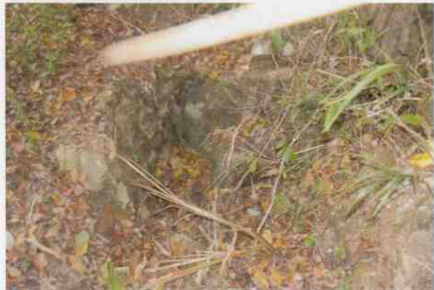
Culvert 15 - Stone kerbing & channelling
