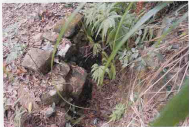
Culvert 51 - U headwall
