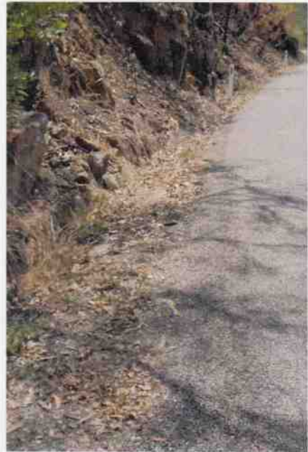
Culvert 153 – Stone kerbing
