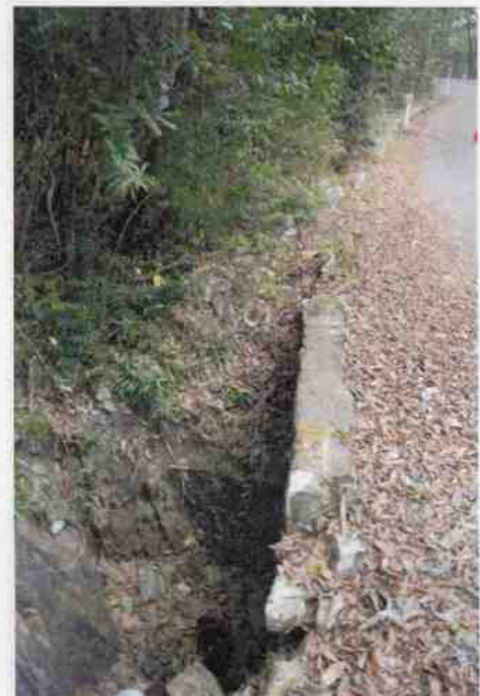
Culvert 34 - Stone kerbing & channelling
