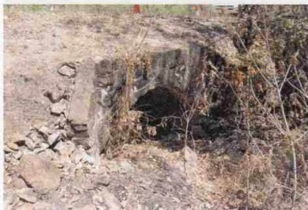
Culvert 210 - E headwall
