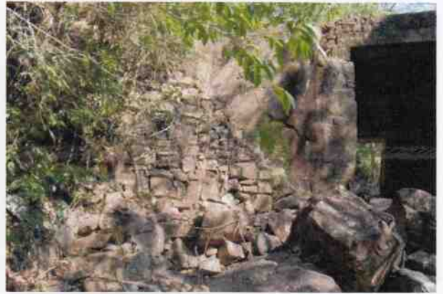
Culvert 141A - E wing wall
