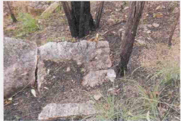
Culvert 206A - Quarry site
