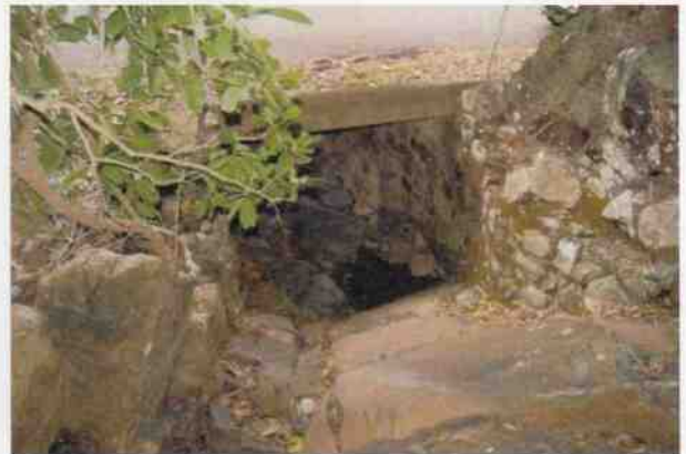
Culvert 98 - U headwall
