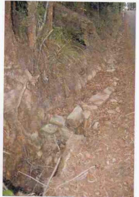
Culvert 70 - Stone kerbing & channelling C091
