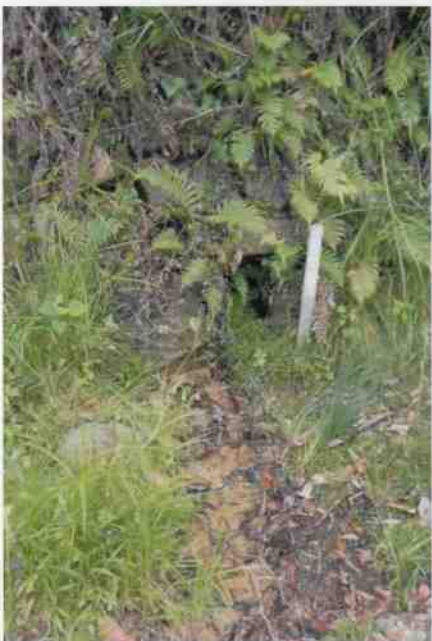
Culvert 95- The Chute water discharge C045
