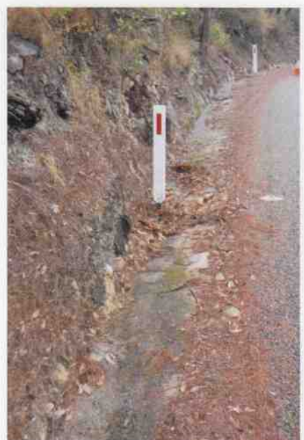
Culvert 126 - Stone kerbing & channelling
