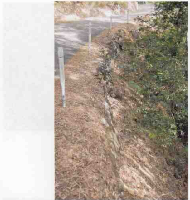
Culvert 62 - E headwall
