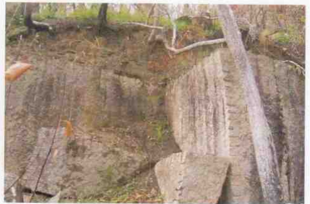
Culvert 206A - Quarry Site
