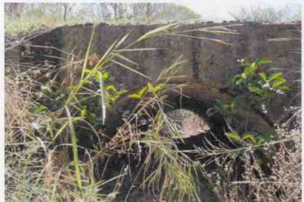
Culvert 210 - U headwall
