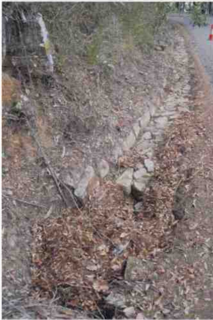
Culvert 69 - Stone kerbing & channelling C093
