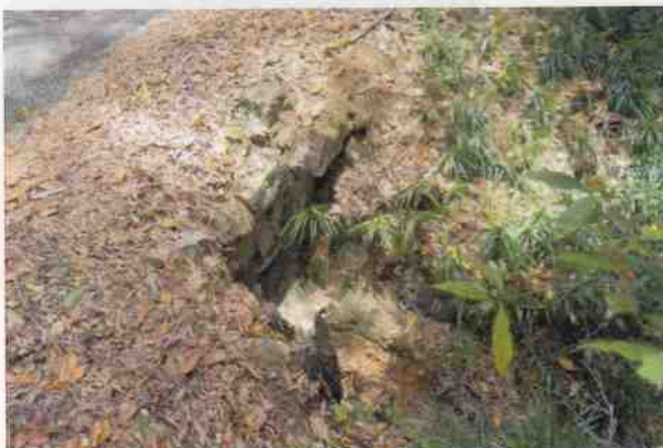
Culvert 43 - E headwall
