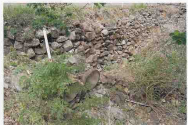
Culvert 94 - Stone retaining wall at E headwall C046
