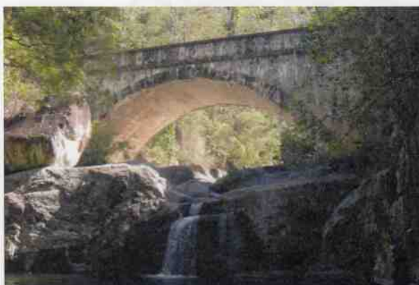
Main bridge C301
