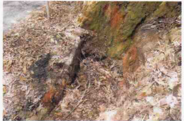
Culvert 38 - U headwall
