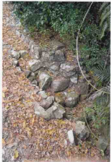
Culvert 8 – Stone kerbing & channelling
