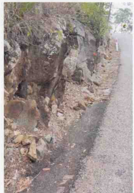
Culvert 112 - Stone kerbing & channelling
