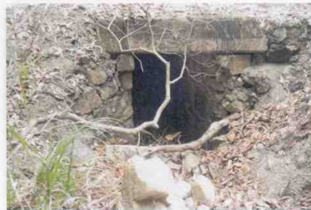
Culvert 45 - U headwall
