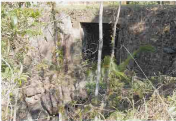
Culvert 141A - Little Crystal Creek carpark B140
