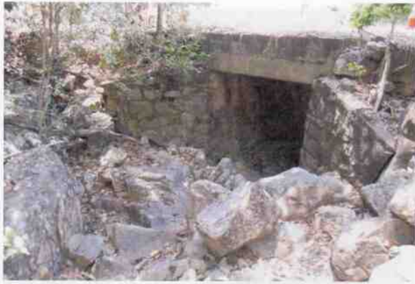
Culvert 150A - U headwall
