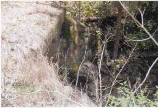
Culvert 87 - E headwall
