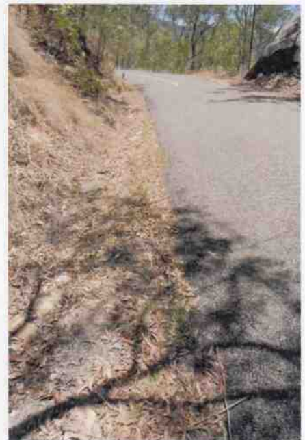
Culvert 201 - intermittent stone channelling
