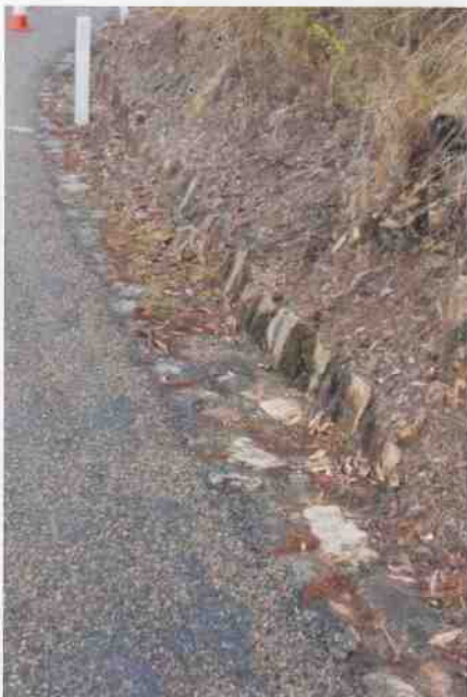
Culvert 123 - Stone kerbing & channelling
