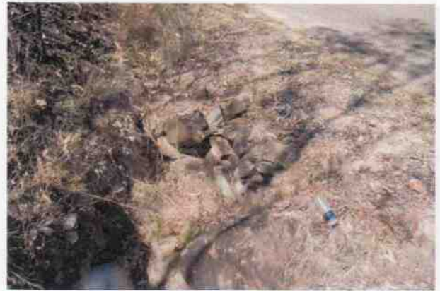
Culvert 216 - U headwall
