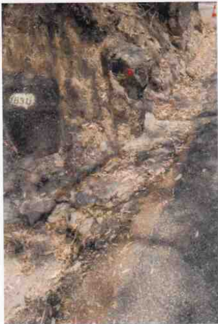
Culvert 163 - Stone kerbing & channelling B102
