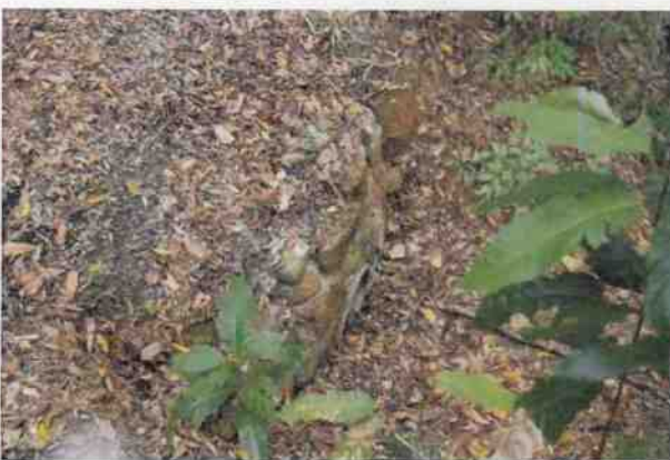
Culvert 37 - E headwall
