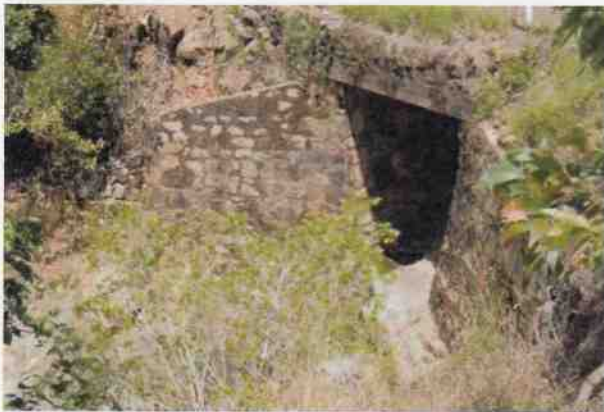
Culvert 150A - E headwall
