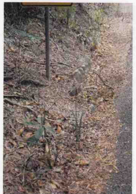
Culvert 3 – Stone kerbing & channelling
