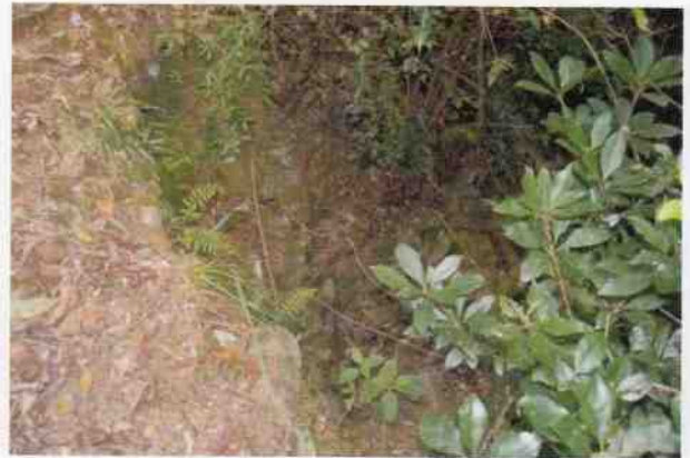
Culvert 31 - E headwall
