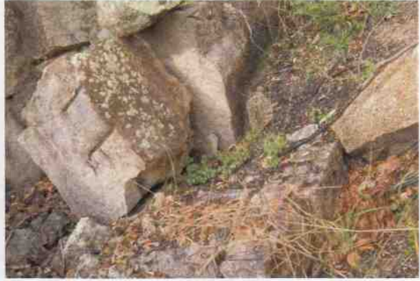
Culvert 206A - Quarry site
