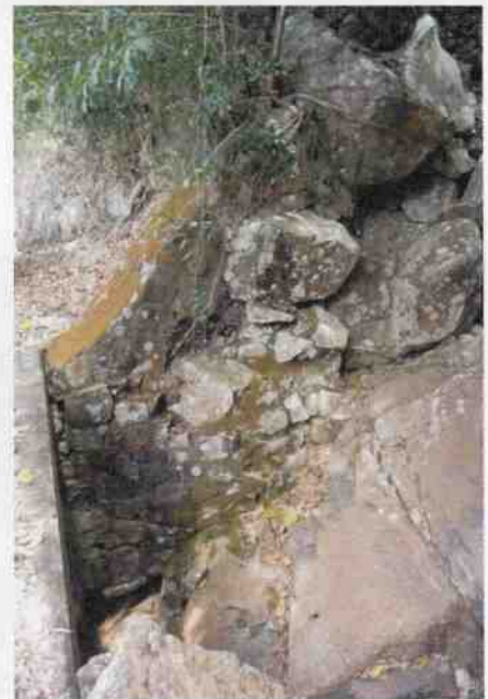
Culvert 87 - Stone training wall
