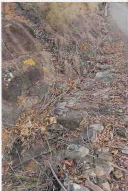
Culvert 115 - Stone kerbing & channelling
