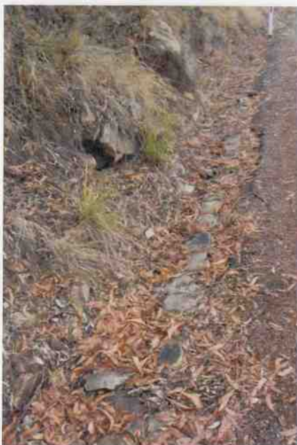
Culvert 117 - Stone kerbing
