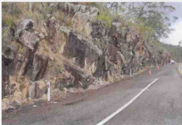
Bartlett's Bluff – large cutting between Culverts 120 and 119
