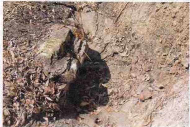
Culvert 149 - Camp site
