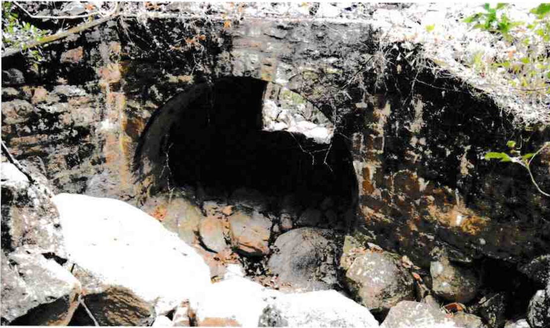
Figure 61 Large culvert headwall constructed in coarsed rubble
