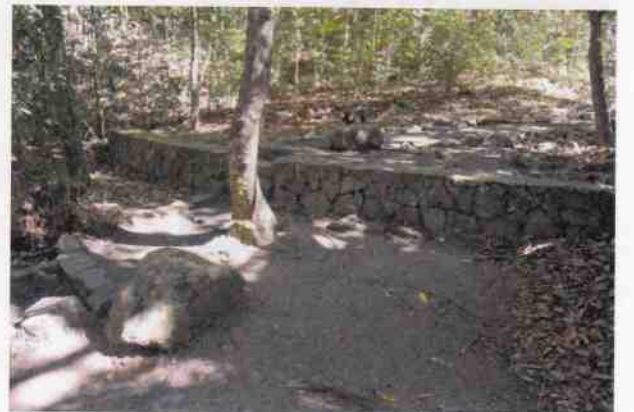
Main bridge - Stone retaining walls to lower picnic area
