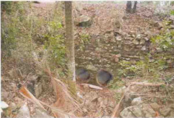
Culvert 106 - U headwall
