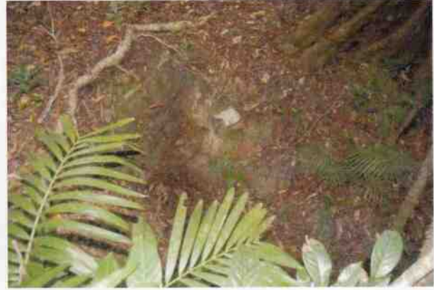
Culvert 22 - E headwall
