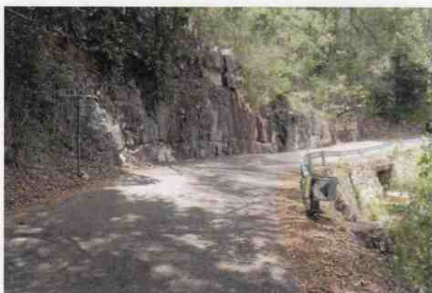
Culvert 40 - Twin Falls
