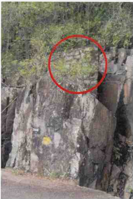
Culvert 40 - Quadrangular training wall above inlets
