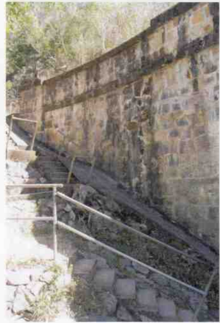
Main bridge – Concrete stairs and path
