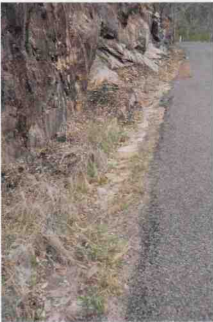
Culvert 176A – Stone kerbing & channelling
