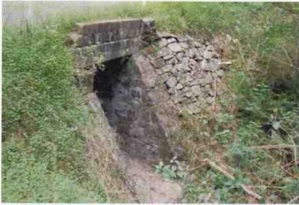
Culvert 55 - E headwall
