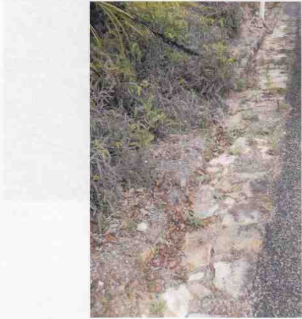
Culvert 15 - Stone kerbing & channelling
