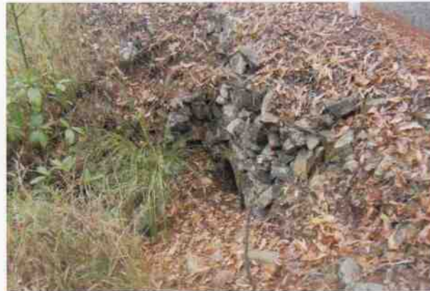
Culvert 132 - U headwall
