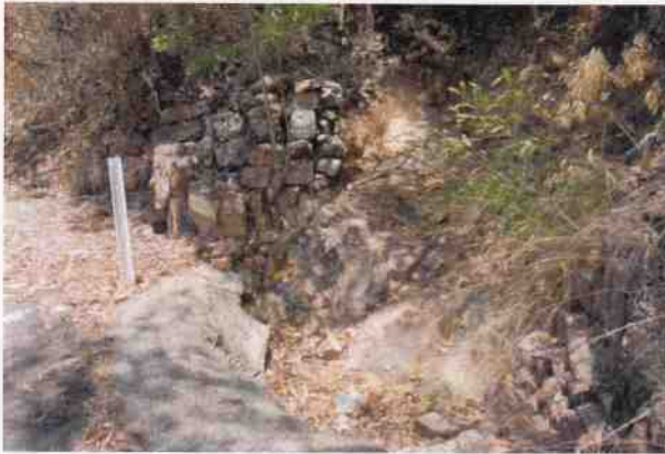
Culvert 157 - Stone wall above inlet
