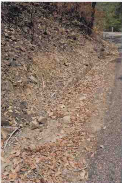
Culvert 151 – Stone kerbing & channelling
